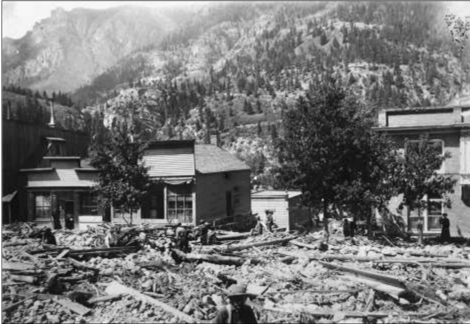
The flood in 1909 pushed Portland Creek over the banks of the channel on the south end of Main Street in Ouray. Similar flooding happened in Cascade Creek on the north end of town. The St. Elmo Hotel is on the right edge of the photo. Photo courtesy of the Ouray Historical Society
