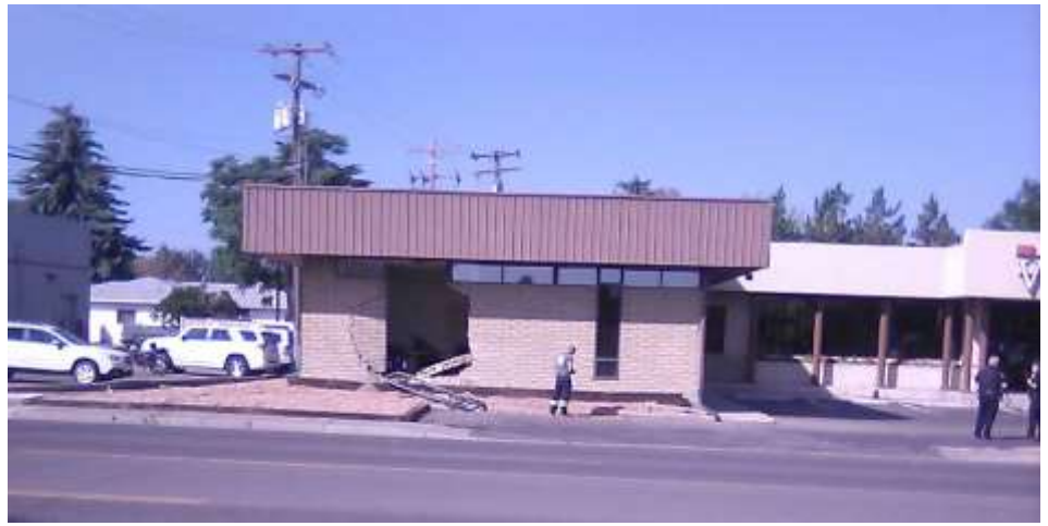
A truck drove through the east wall at Vectra Bank last Monday. Photo by Debbie Blanchard.
