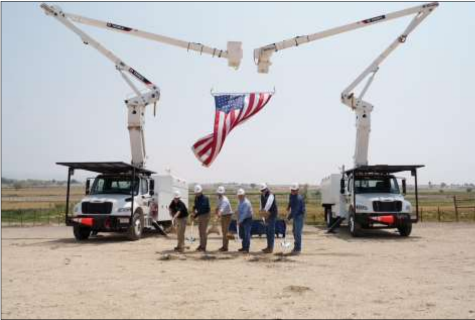
Tuesday, July 23, marked the much-anticipated groundbreaking for Garnet Mesa Solar. DMEA Courtesy photo.
