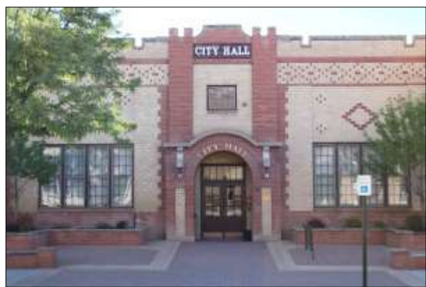
Historic City Hall Building. Photo by Harry Switzer
